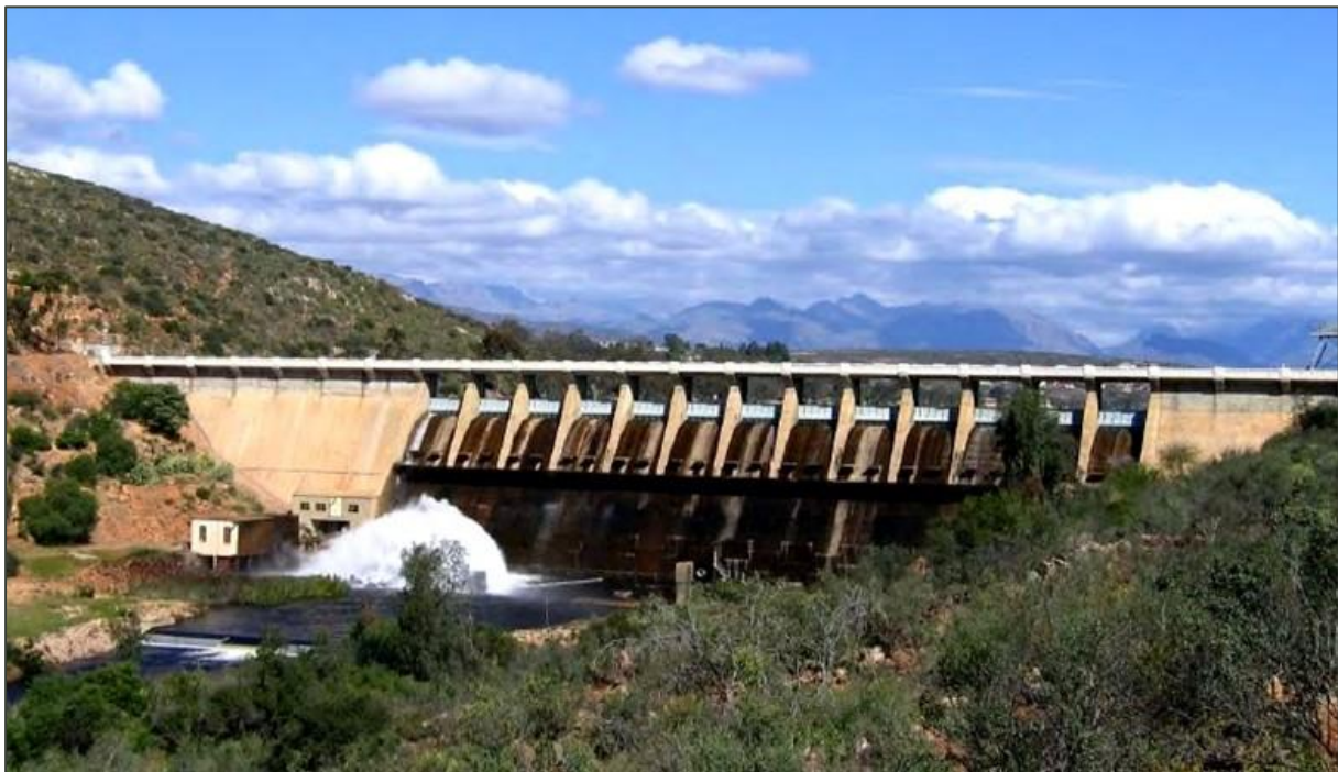
Figure 1-1: Clanwilliam Dam Photo courtesy of DWS
