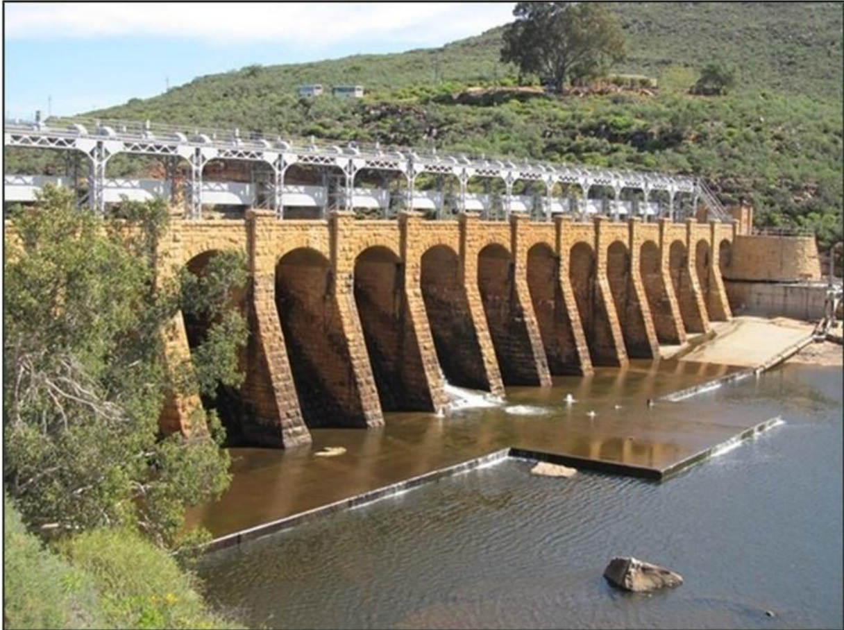
Figure 7-3: Concrete masonry Bulshoek Weir
