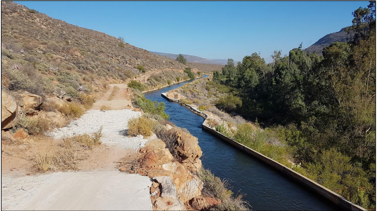
Figure 7-9: Existing Left Bank Canal looking downstream (approx. ch. 1.2 km)
